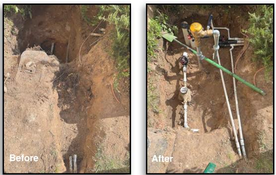
above and then back below the irrigation lines. As the roots have grown, they exert pressure on the bends in the pipes and have, or soon will, cause breaks. These breaks tend to be at connection points.
