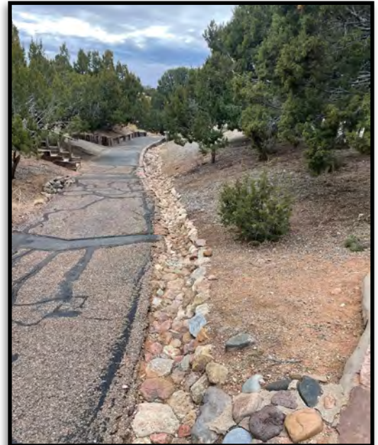
Closer view of the drainage ditch
