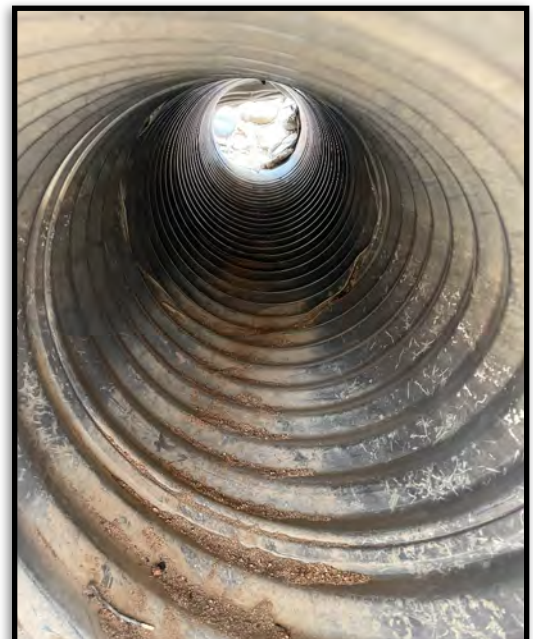
Unblocked culvert
